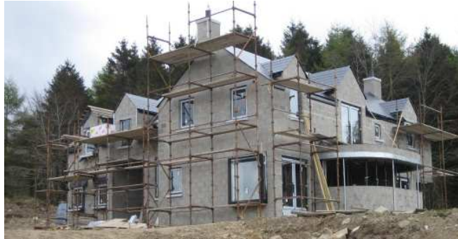
Front of Dwelling During Construction
