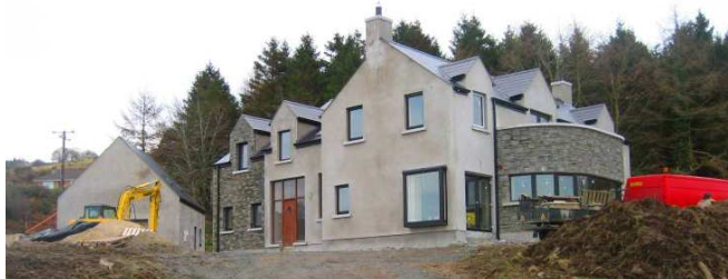
Front of Dwelling Nearing Construction
