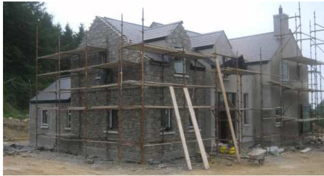
Side of Dwelling During Construction
