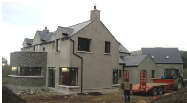
Side of Dwelling Nearing Completion
