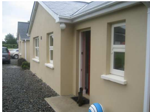
Front & Side of Dwelling After Extension
